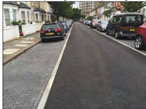
Permeable paving beneath parking
